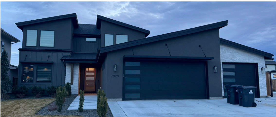
Modern exterior, mono-sloped roof with multiple roof breaks
