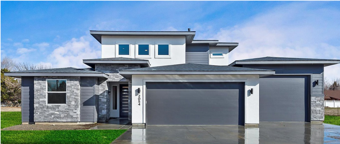
Minimalist exterior with multiple roof breaks on a low profile roof
