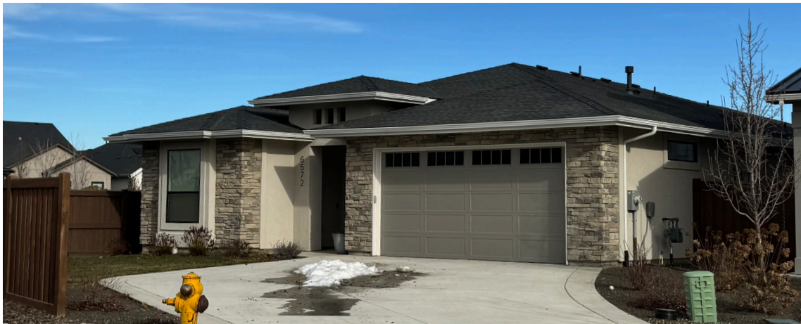
Example of too much roof facing the street and lacking roof breaks ( not permitted )
